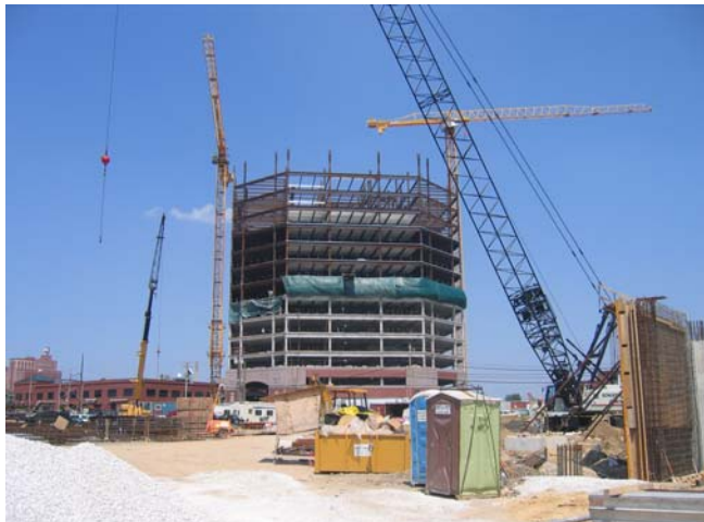
Fig 4 – Steel & Precast Erection with a view of fireproofing plastic
