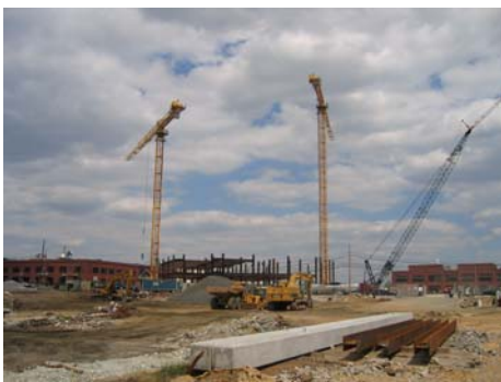
Fig 10 – Tower cranes from afar
