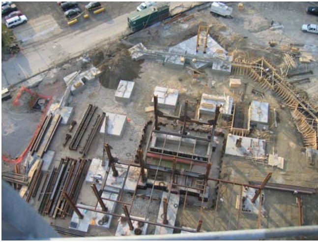
Fig 8 – Aerial view showing poured pile caps and beginning of column erection
