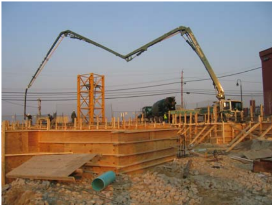
Fig 15 – Concrete Pump during foundation pours
