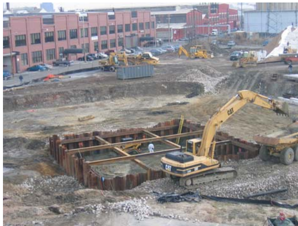
Fig 17 – Shoring for elevator pits
